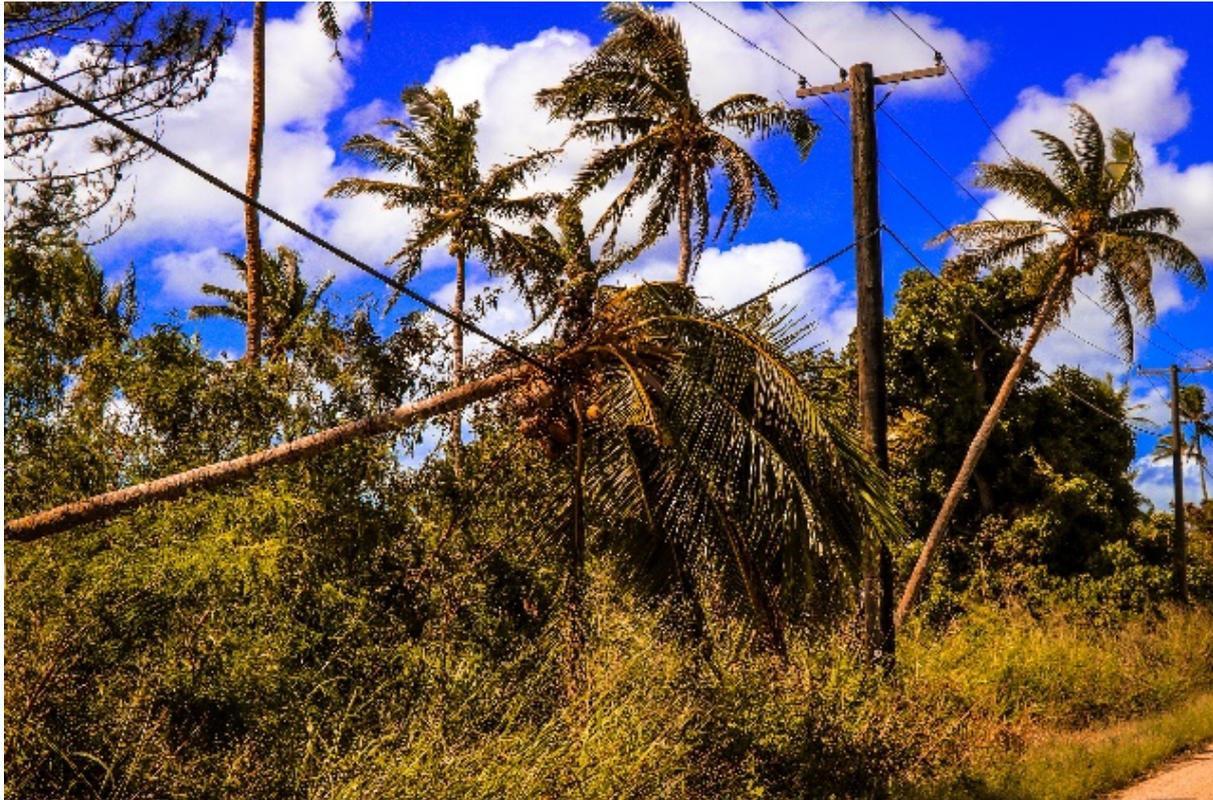
Figure 5 An example of LV ABC conductor resilience to tree damage during a cyclone.
